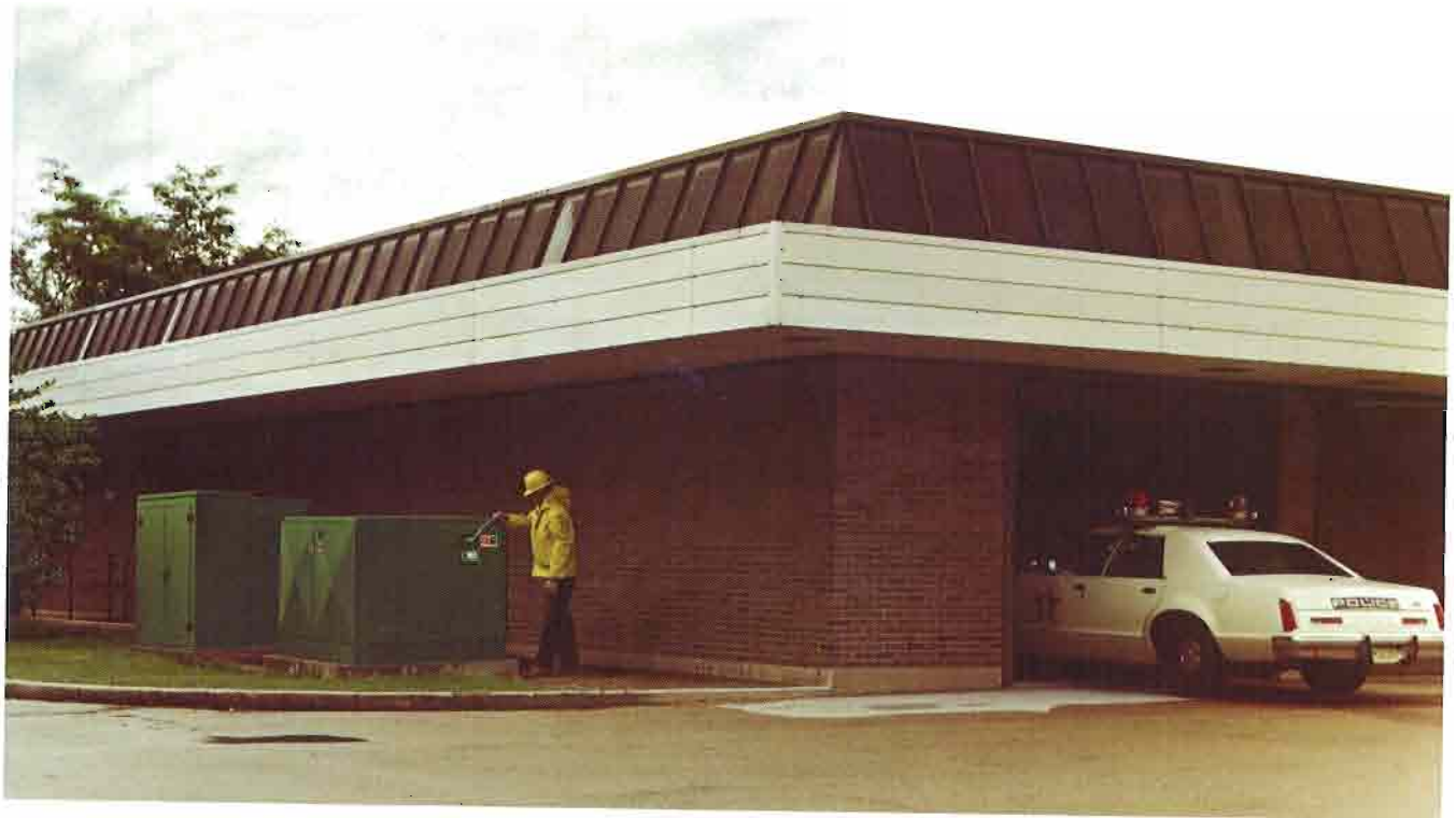
Figure 4. The PMH-6 pictured above provides primary-selective service in this institutional application.
