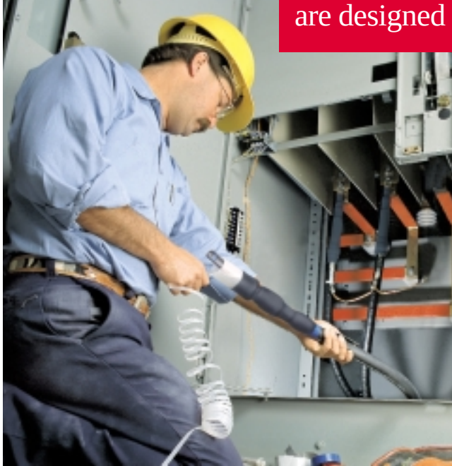
Cold Shrink QT-III Indoor Termination
